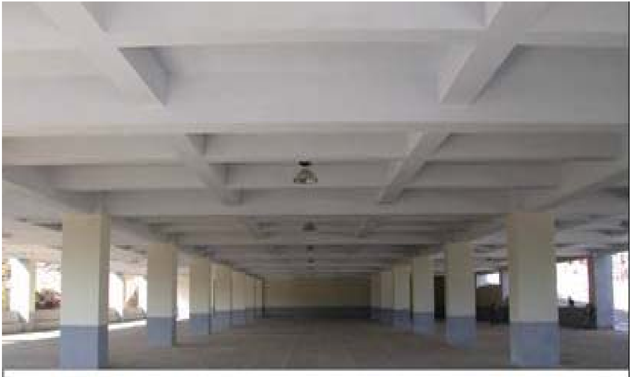
INNER VIEW - HEAVY VEAVY VEHICLES PARKING KHLIEH IEWDUH, SHILLONG
